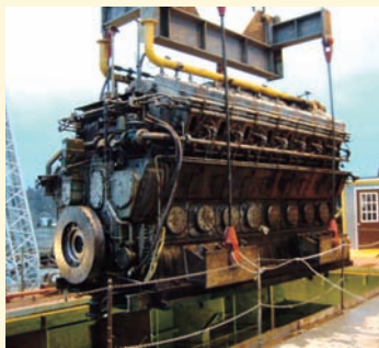
Out with the old (above) and in with the new (right) for the Edwin H. Gott .
