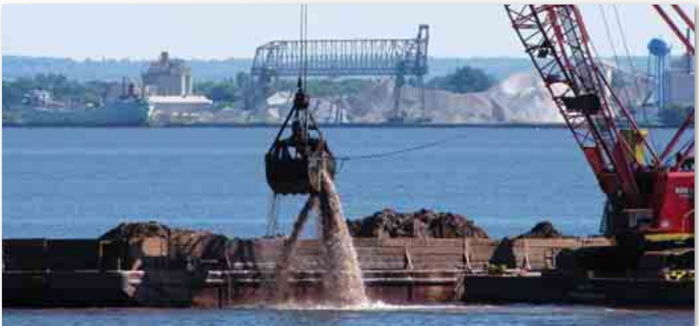
A clam-shell bucket — just part of the gear that is deployed in the 21st Avenue West pilot project — takes a big bite out of the harbor.
