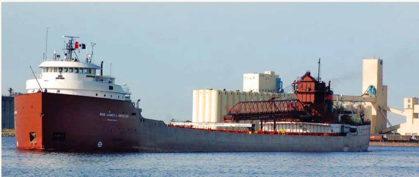
Interlake Steamship Co. is one of many companies exploring scrubber systems to comply with ECA standards. During winter layup, two exhaust gas scrubbers are being installed aboard its Hon. James L. Oberstar .
