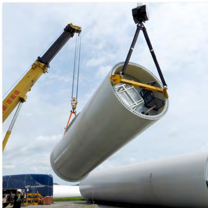
The lifting beam and rigging at work here are what distinguish Duluth's LiftPRO.
