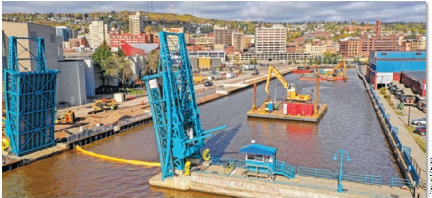
As soon as the Irvin moved out, crews from J. F. Brennan moved in and began the process of capping legacy contaminants.
