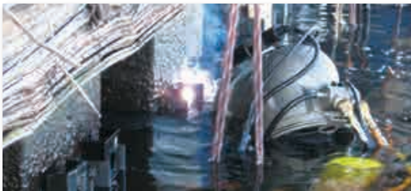
The new company's staff is hard-hat trained and certified.
