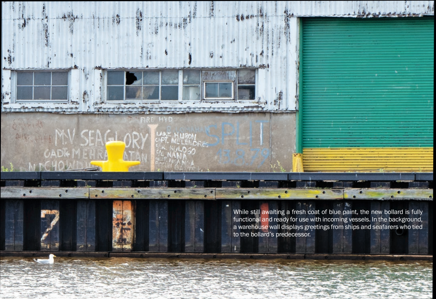
A bollard secures a vessel at berth. Multiple bollards are used in this process to ensure that the ship stays in place during the loading and unloading process and in the event of strong weather.
