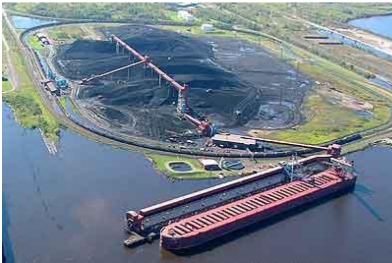
The Midwest Energy Resources Company's Superior terminal, a showpiece of Great Lakes port development, continues to set port coal-handling records. (Duluth Shipping News Photo)
